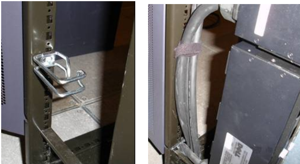
Figure 7 – Remove cord guides (leftmost picture) and secure PDU inlet cords to the rack by tie wraps or hook and loop fastener straps.
