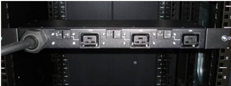
Figure 6 - Mounting of PDU inside the U-Space using adapter kit provided with PDU.
