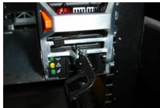
Figure 10d - Power cord removed
